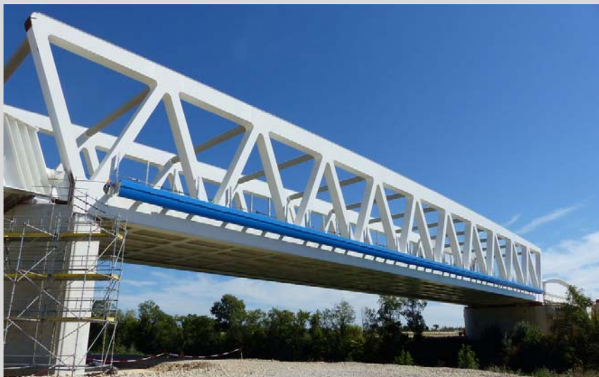
Ouvrage SC 581 Vidourle - © SAPB
